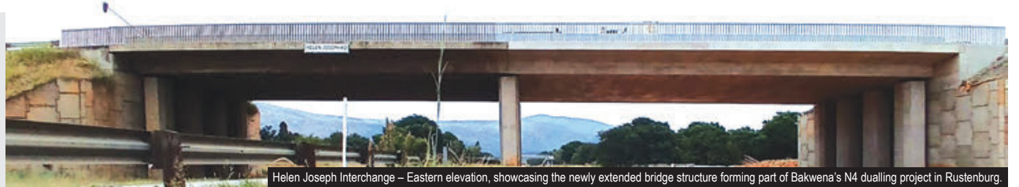
Helen Joseph Interchange – Eastern elevation, showcasing the newly extended bridge structure forming part of Bakwena’s N4 dualling project in Rustenburg.
