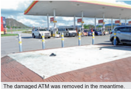
The damaged ATM was removed in the meantime.
